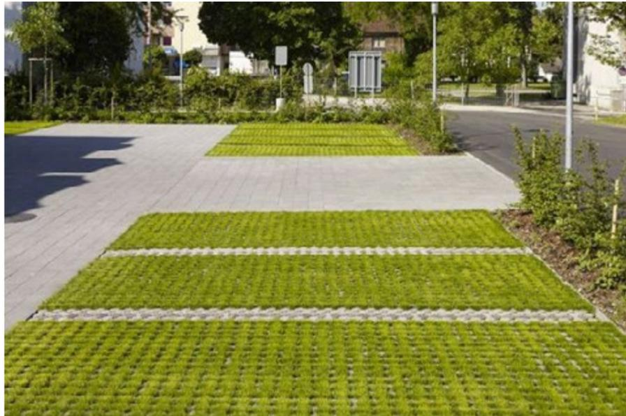
Permeable paving solutions used where appropriate in parking areas and emergency access route.
